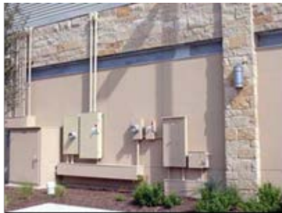
Utility equipment at back of building painted to match wall
